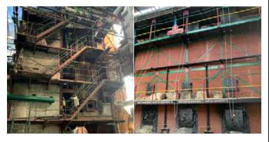
Figure 1 - Bagasse fired water tube Boiler; Make - Walchandnagar Industries.
