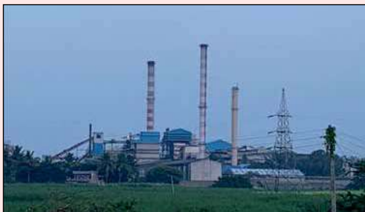
[Photo 1 – Typical sugar industry with Co-gen plant – Early morning view]
